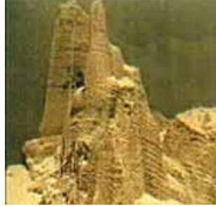
View of soya build up from down inside silo just prior to activation of one Cardox Tube.
